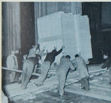
The photo shows the case containing the Pietà being led gently down a ramp through the portico of the Basilica.
