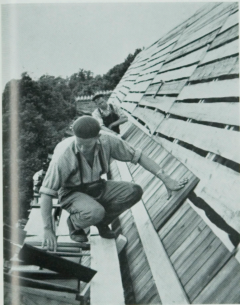
The shingles are laid
