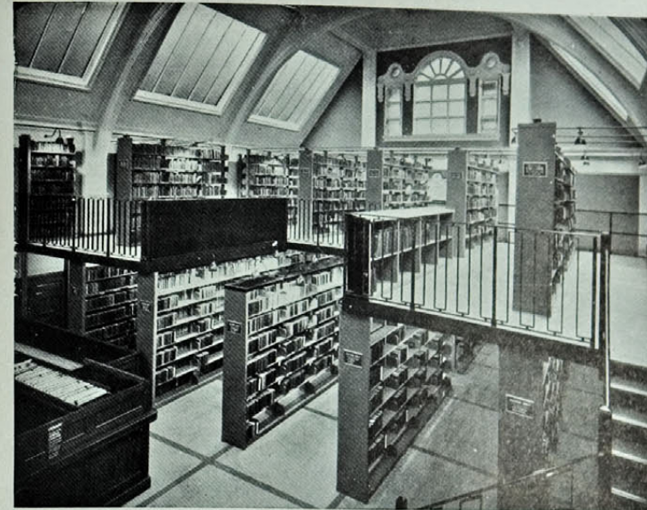
Central Library, Walthamstow
